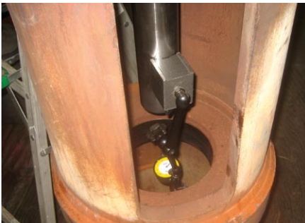
CV crosshead bushing sweep to assure concentricity following corrective action.
